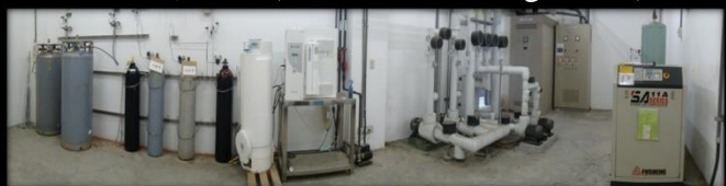
管道間(Facility Room)
