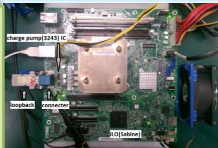
Fig. 2 The failure main board
